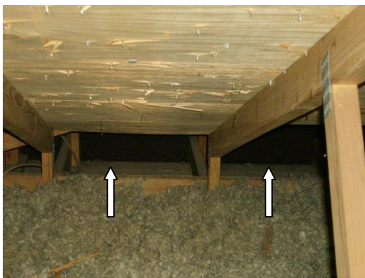
Missing Insulation
